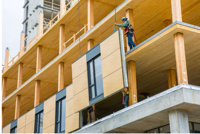
Figure 6: Brock Commons Tall wood House, a residence building where cross laminated timber has been implemented. (Naturally: wood, 2017)
