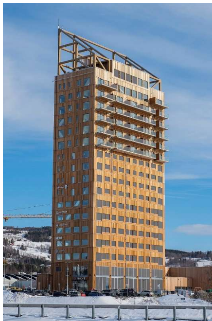
Figure 5: The Lake Mjøsa Skyscraper in Brumunddal, Norway, which is built of cross-laminated timber (CLT). (Øyvind Holmstad, 2019)
